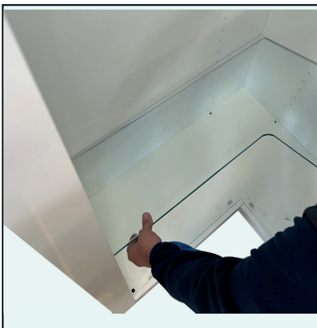
7. Place the first shelf, starting from the bottom.
